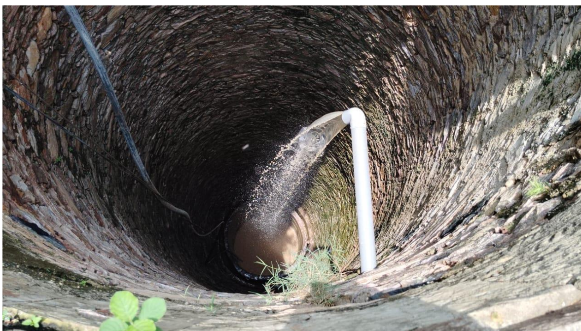
A completed and recharged open well showing significantly improved water depth — Kotkhawda block
