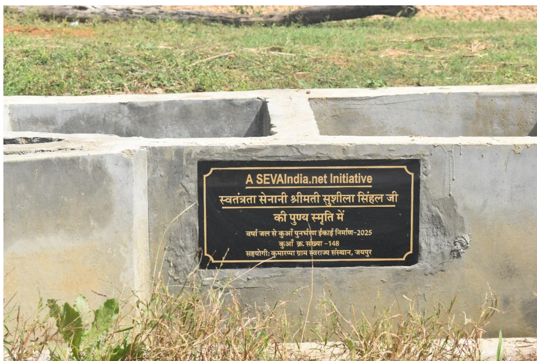
Well Recharge Structure
