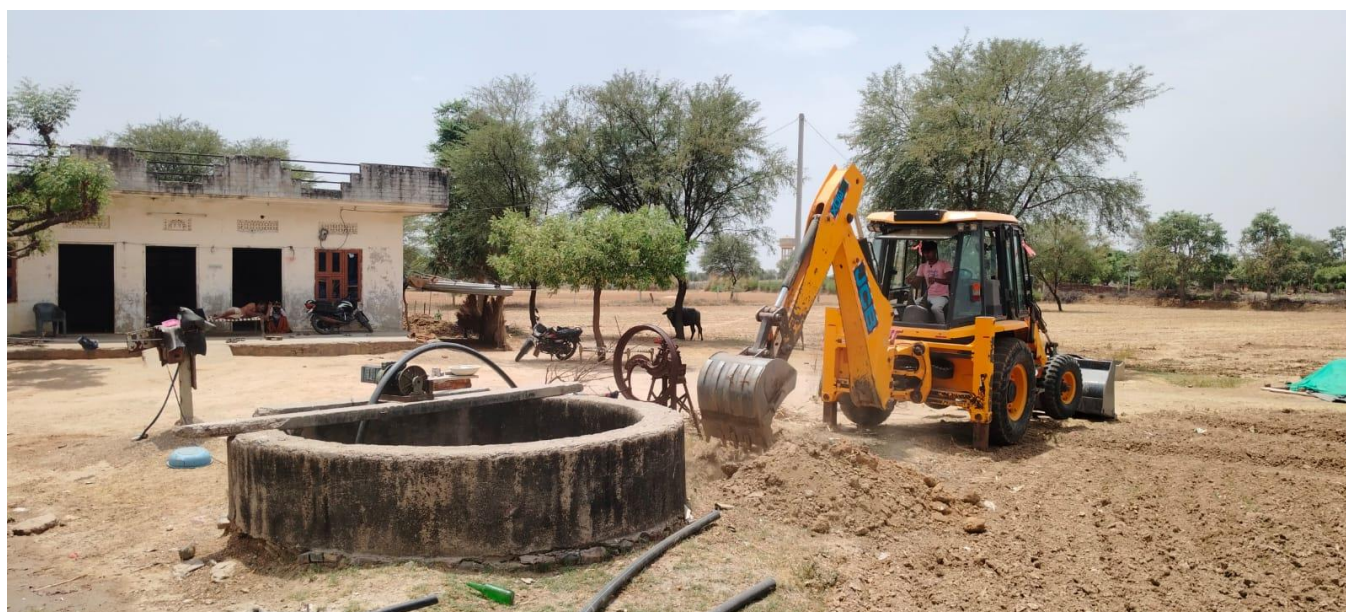
Pipeline laying work in progress during construction of a well recharge structure — Kotkhawda block
